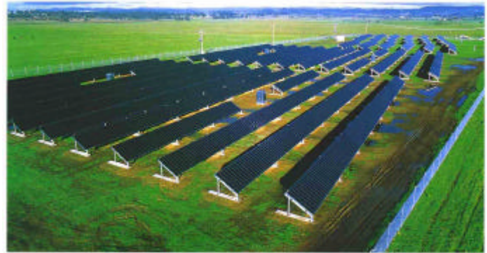
Figure 4: Singleton (NSW) solar farm (Photo courtesy energy Australia)
